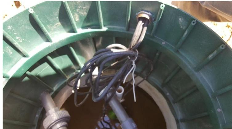
All wiring connection at the tanks will be made inside of this sealed box. Once the wiring connections have been made, a sealant is used to prevent sewer gas from entering the electrical connections. Water proof type wire nuts are used to connect the 3 floats and 2 pumps.
