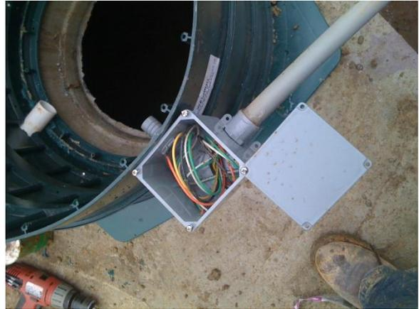
The 12-3 wire and irrigation 7 lead wire should be fed through the waterproof connectors in the bottom of the grey electrical connection box at the pump tank.
